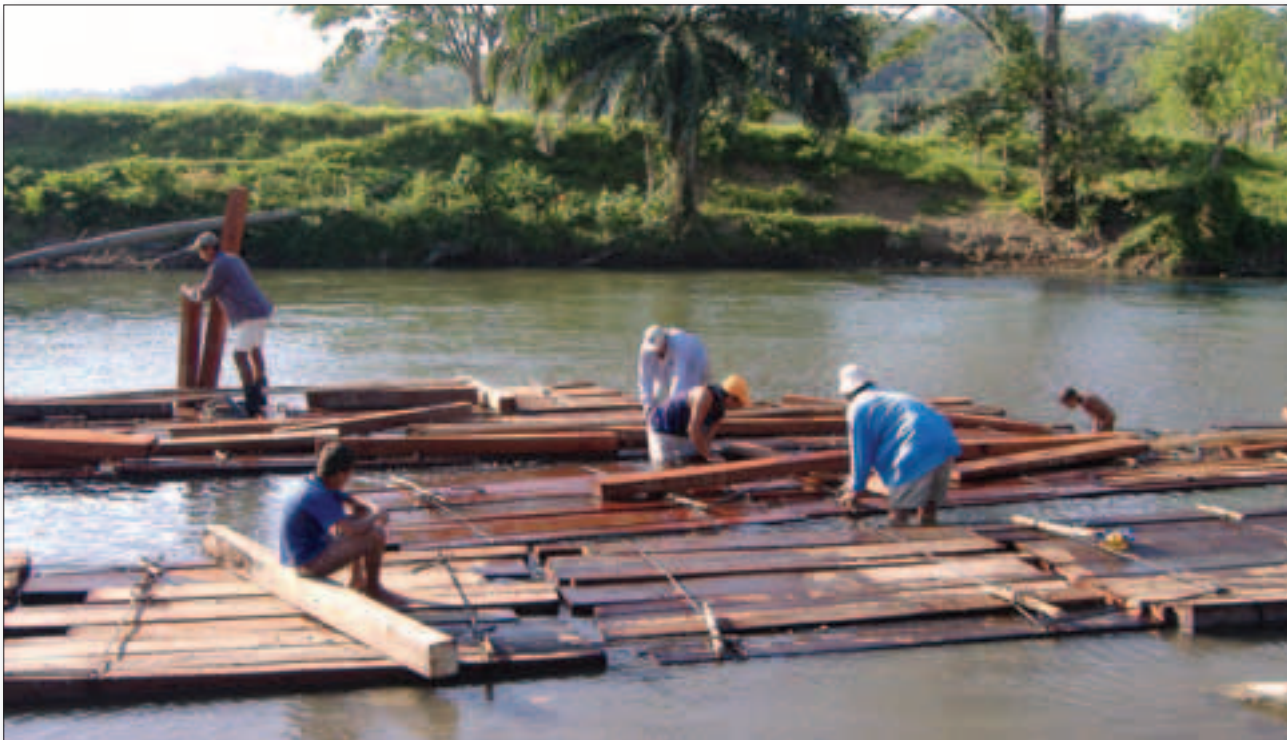
Constructing timber rafts before floating them downriver
