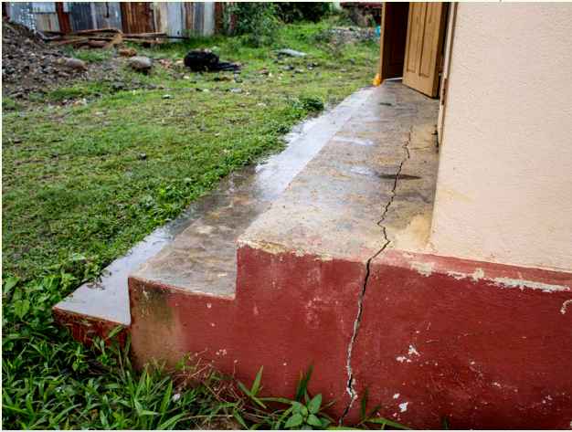
Cracks in one of the Kaday monastery buildings which the monks blame on the violence of the jade mining operations in the crater below. CREDIT: Minzayar
