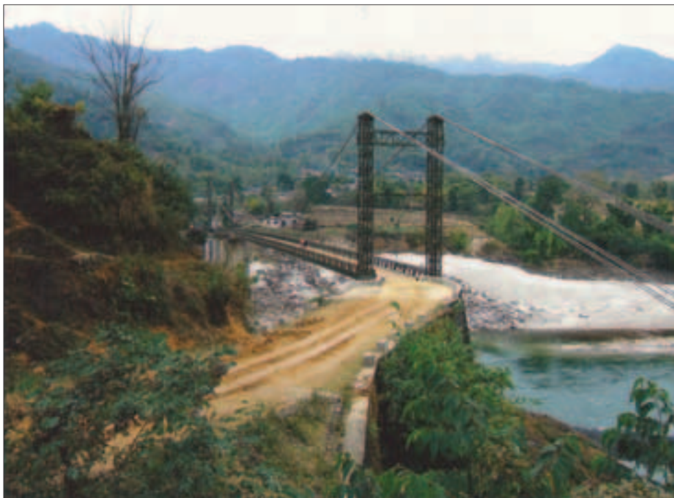
The Chipwe Bridge
