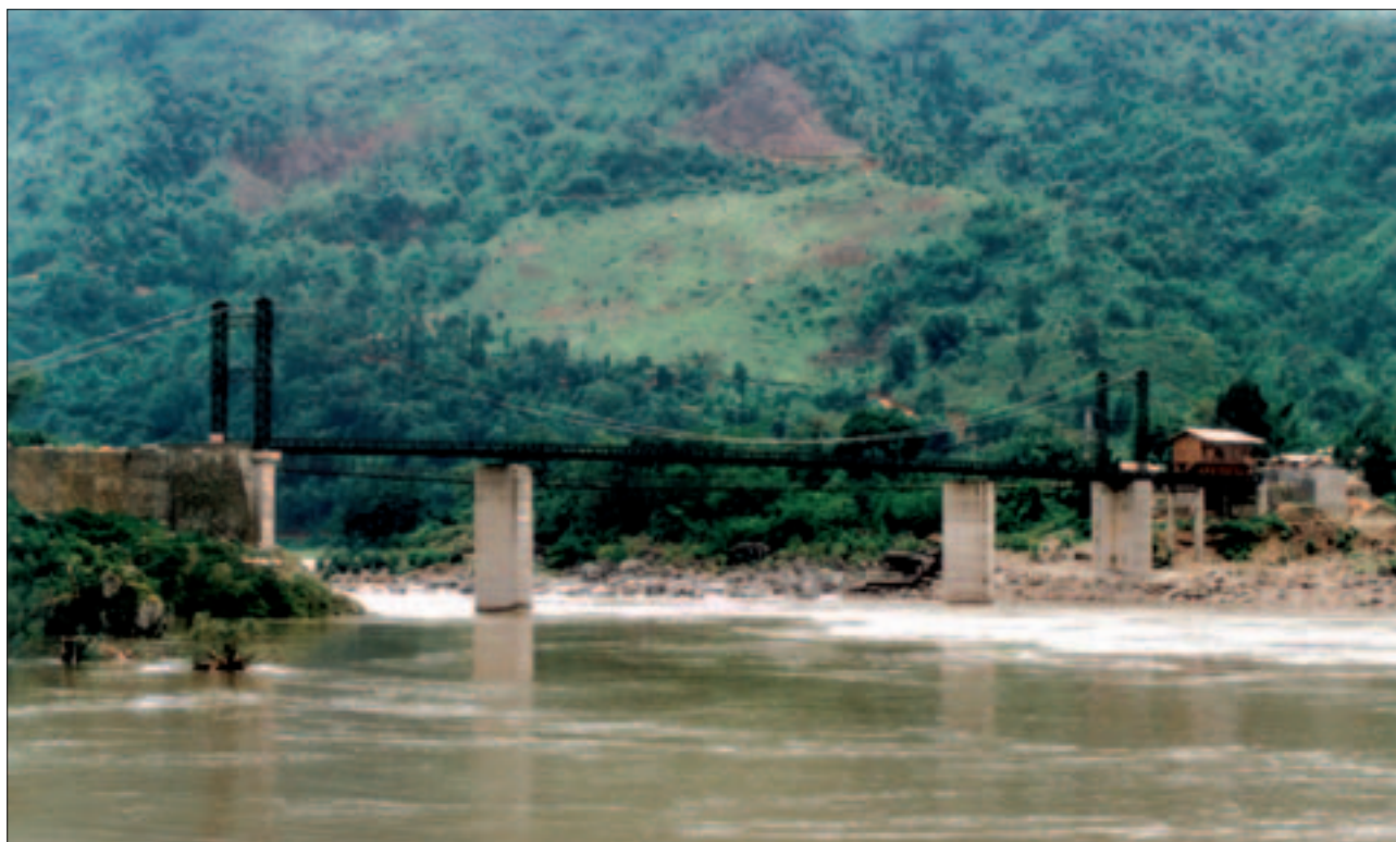
The new Chipwe Bridge which opened in March 2004
